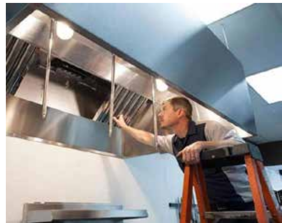
Figure 2: Manual Inspection of the Kitchen Hood [2]
