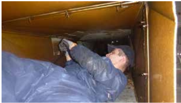
Figure 1: Manual Scraping of the Ducts[1]
